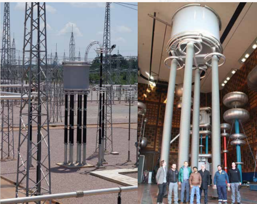
HVDC Smoothing Reactor (600 kV on the left / 800 kV on the right)
