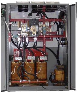
Redundant chargers with common battery compartment
