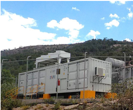
Mining 6 MVAR STATCOM
