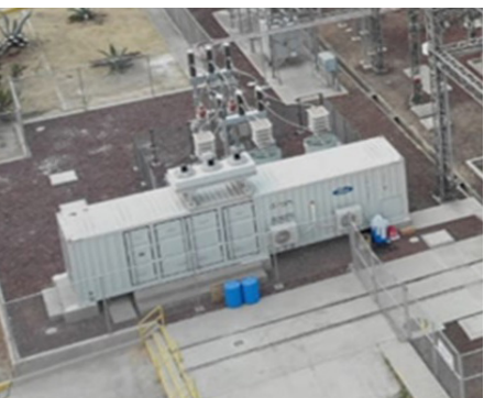
Automotive 4 MVAR STATCOM
