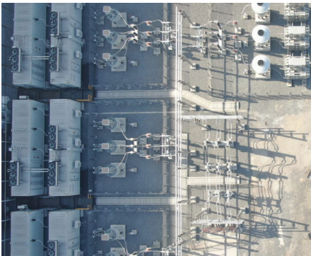
Steel (EAF) 320 MVAR STATCOM
