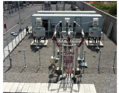
Steel (EAF) 40 MVAR STATCOM
