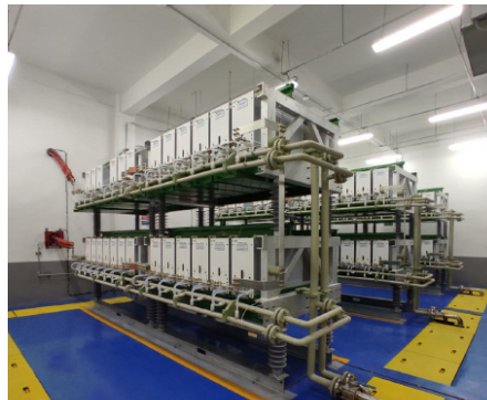
Steel (EAF) 120 MVAR STATCOM
